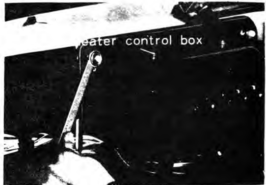
Fig. 13-23 Removing heater control box
