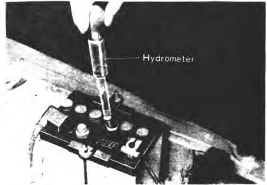
Fig. 2-3 Measuring specific gravity of battery electrolyte
