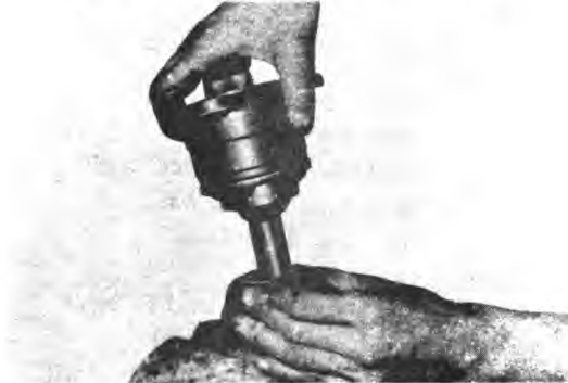
Fig. 4-45 Inserting outer race
