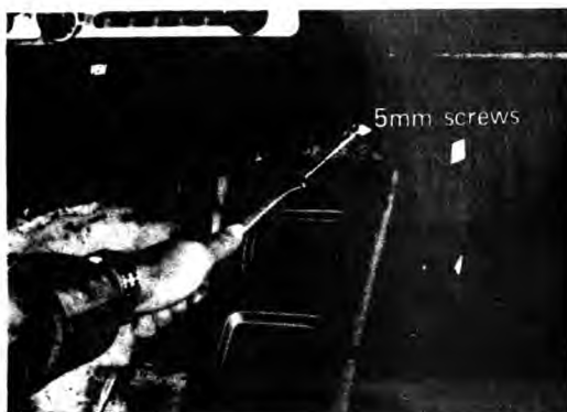
Fig. 7-8 Removing inspection cover
